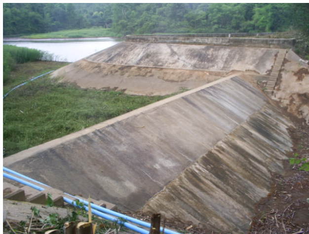
Heightening the spillway's embankment by one metre
