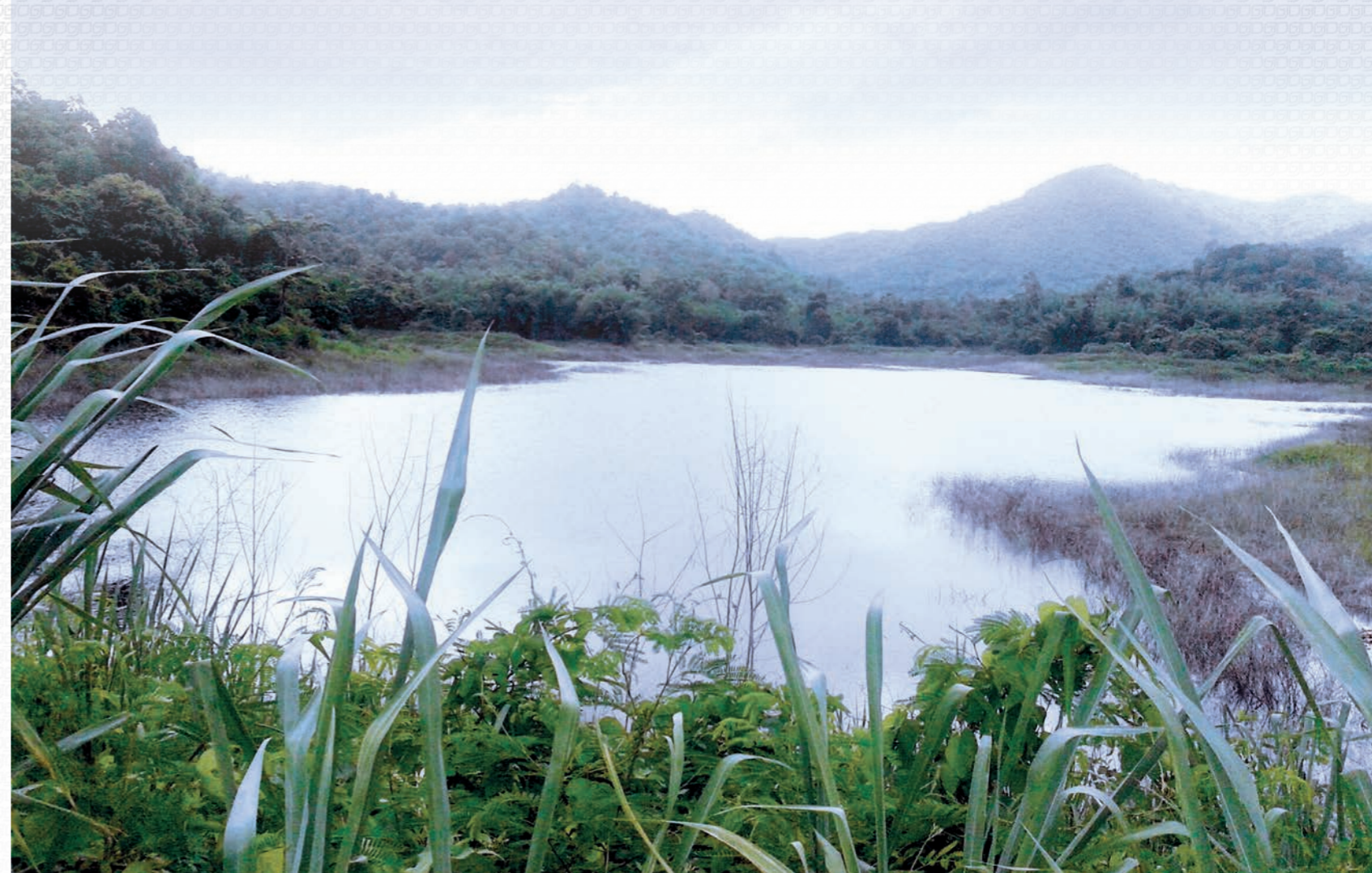
5. The Royal-initiated Upper Hin Si Reservoir in Village No. 4, Yang Hak Subdistrict, Pak Tho District, Ratchaburi Province, was constructed with its earthen embankment which is six metres wide, 240 metres long, and 21 metres high. With an 8.25-square-kilometre area to retain rainfall, it has a capacity to hold 1,064,000 cubic metres of water.
