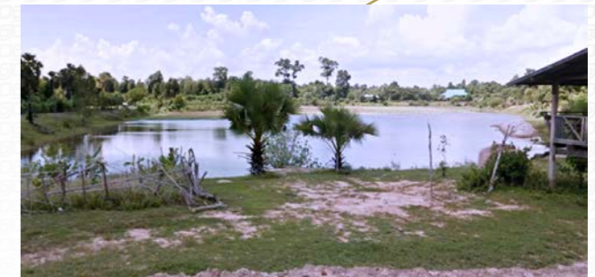
The Nong Mek Swamp of about 5.6 hectares (35 rai) was dredged, with its embankment being reinforced via levelling and compaction techniques.
