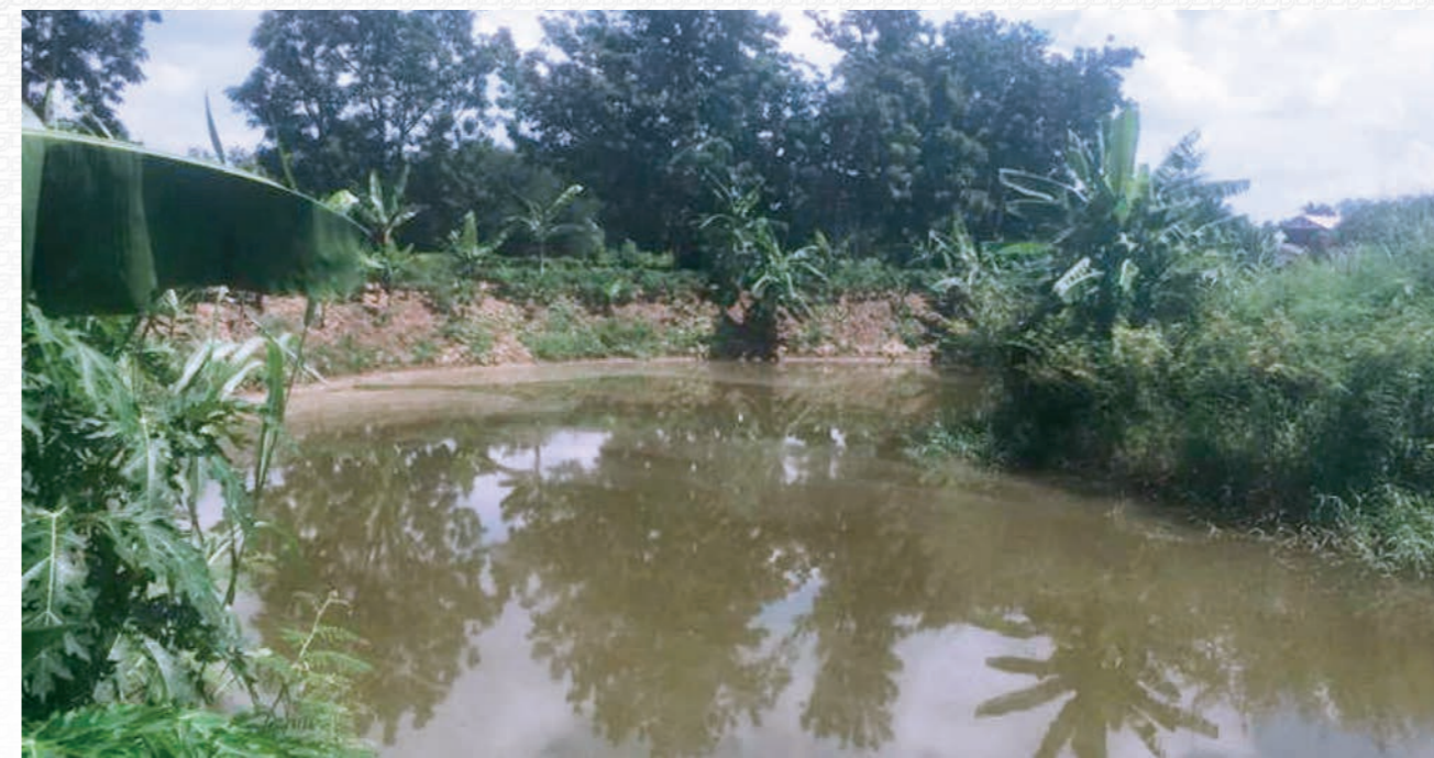
The canal dredging in Village No. 14 renders benefits to 80 hectares (500 rai) of land.
