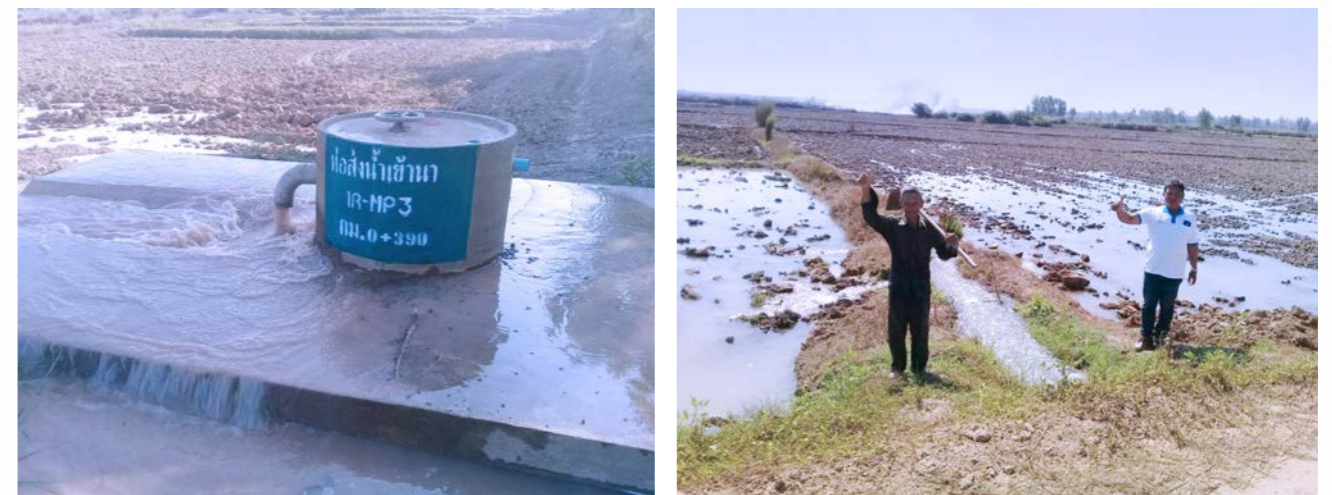
The area of the project after its completion in 2018
