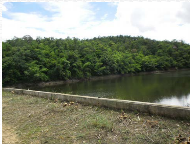
Raising the height of the earthen embankment in the upstream section by about one more metre to ensure it could safely handle any fast-rising water level
