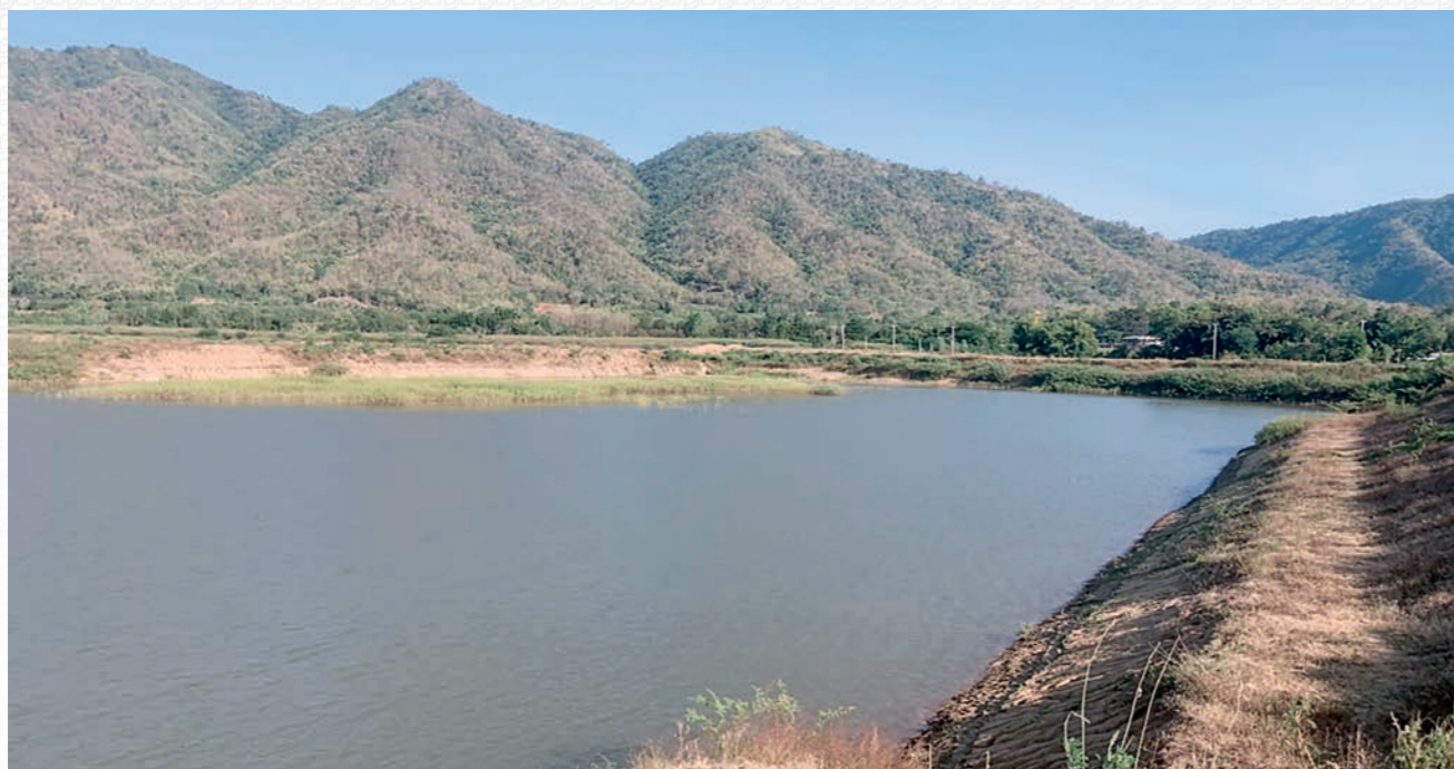
Huai Yai Monkey Cheek with its water-retaining capacity of 373,000 cubic metres
