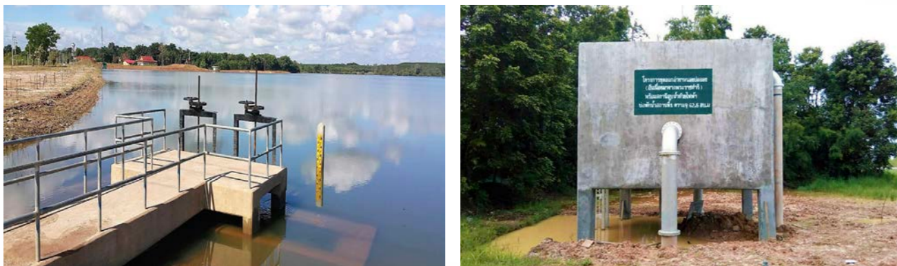
The area of the project after its completion in 2018
