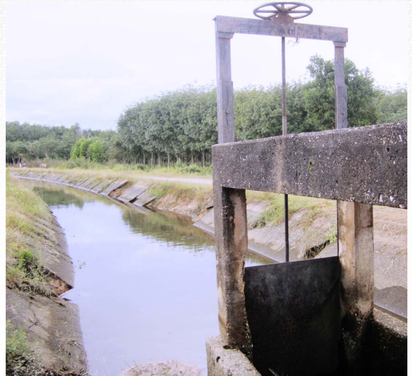
A construction of a water distribution canal system for Ban Ku Bae Si Ra Village
