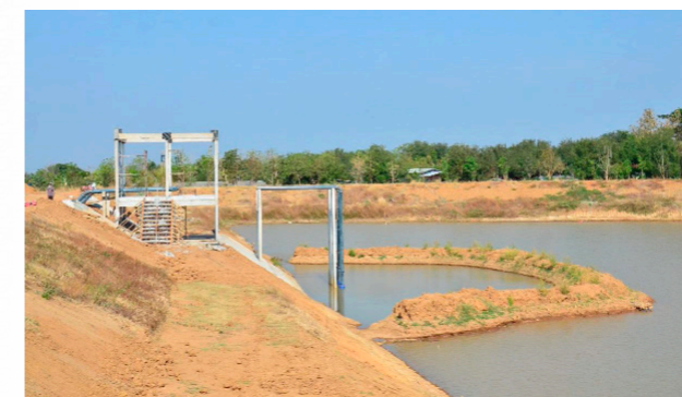
The Ban Huai Haen Electric Water Pumping Station
