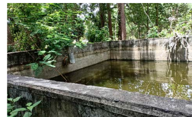
A reinforced concrete sedimentation pond
