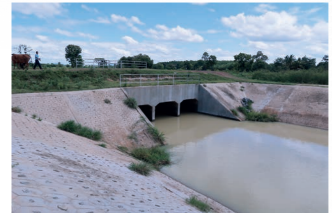
The creek, after being dredged, becomes 20 metres wide, 2,905 metres long, and 4 metres deep, equipped with sluice gates.
