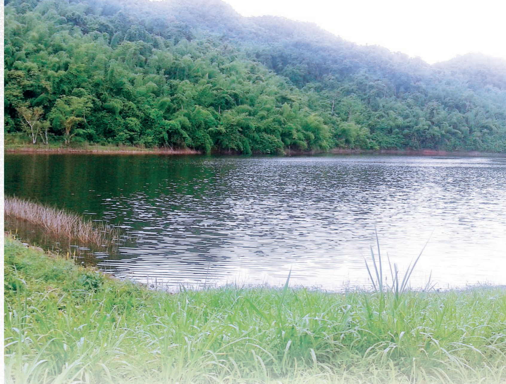
3. The Royal-initiated Khao Hua Daeng Reservoir in Village No. 3, Yang Hak Subdistrict, Pak Tho District, Ratchaburi Province, was constructed with its earthen embankment which is six metres wide, 180 metres long, and ten metres high. With a 7-square-kilometre area to retain rainfall, it has a capacity to hold 612,000 cubic metres of water.
