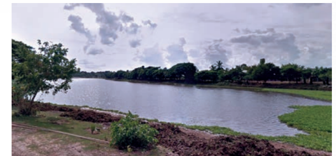
The Nong Bua Dong Swamp of about 31.68 hectares (198 rai) was dredged, with a gravel road being constructed nearby.
