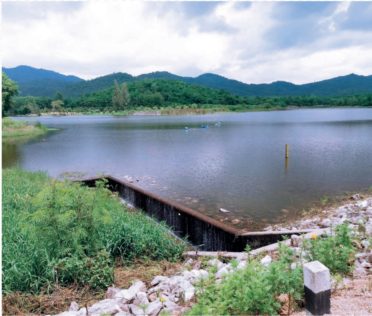
2. The Royal-initiated Huai Phu Krut Reservoir in Village No. 4, Yang Hak Subdistrict, Pak Tho District, Ratchaburi Province, was constructed with its earthen embankment which is five metres wide, 326 metres long, and 13 metres high. With a 10-square-kilometre area to retain rainfall, it has a capacity to hold 270,750 cubic metres of water.
