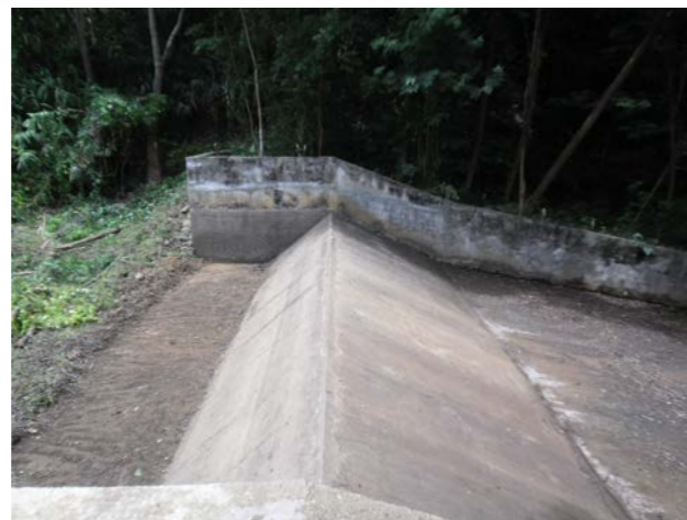
Increasing the height of spillway by one more metre
