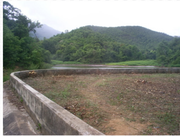
Heightening the upstream embankment of the earthen structure by 1.1 metres higher than before
