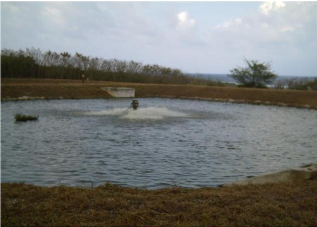
Fig. 3. At the Inarajan Sewage Treatment Plant each cell is aerated by floating mechanical surface of aerators running daily for 24 hours.
