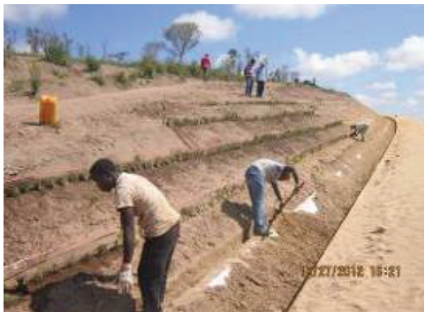
Photo 17, 18 Slope stabilization of National Highway No. 1, the Republic of Congo
