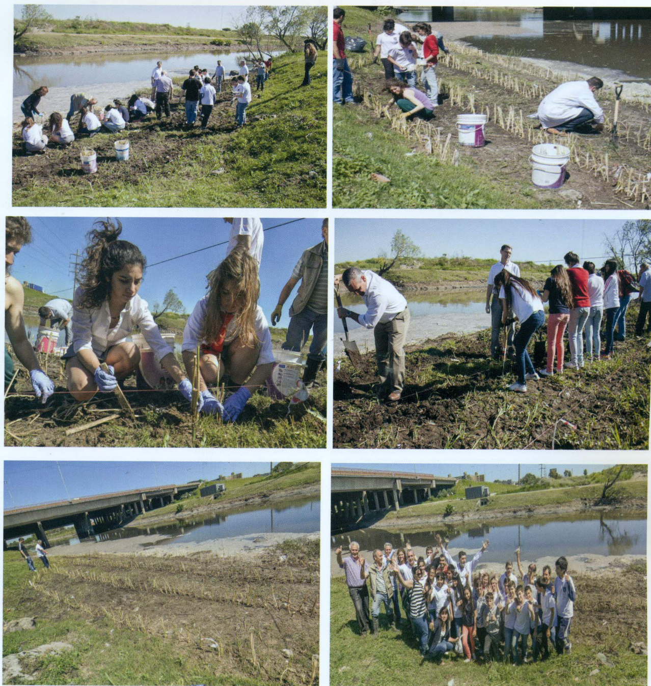
Planting 1000 vetiver tillers to remediate the bank of Arroyo Sarandi River, Buenos Aires
