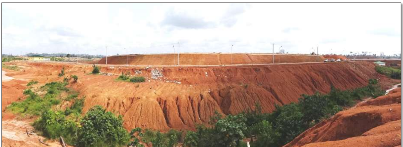
Before & After VST Application for Slope Stabilisation – Reasonable cover attained on slopes PC
