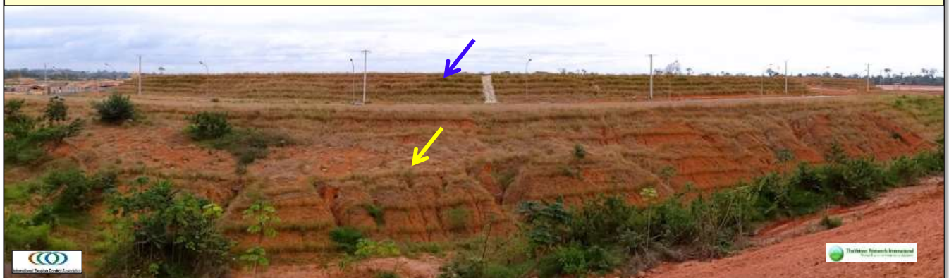
Before & After VST Application for Slope Stabilisation – Reasonable cover attained on slopes PC
