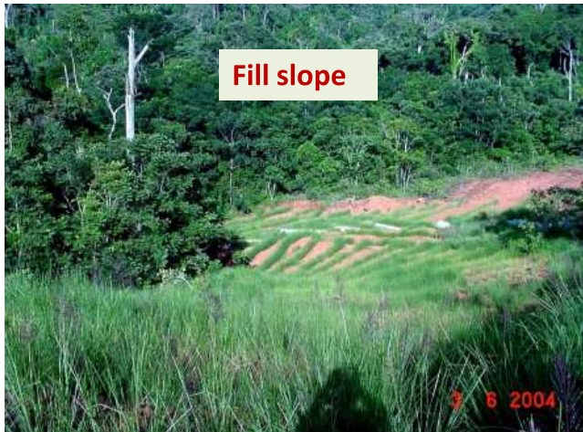
VST for erosion and sedimentation control at Los Pijiguaos Bauxite mine
