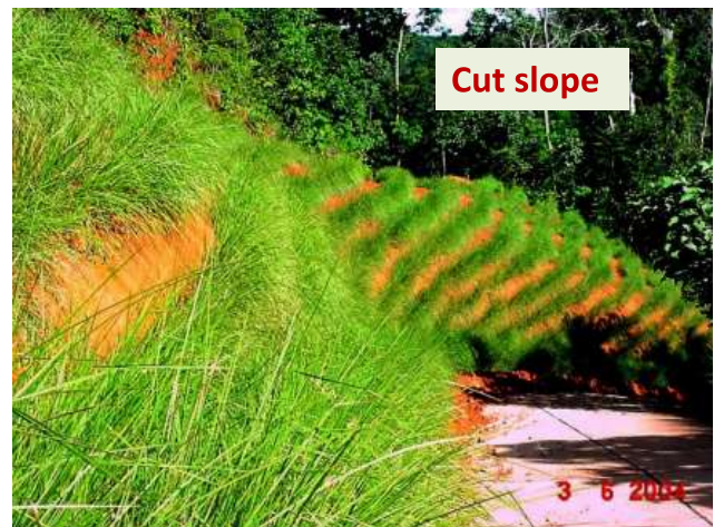
VST for erosion and sedimentation control at Los Pijiguaos Bauxite mine
