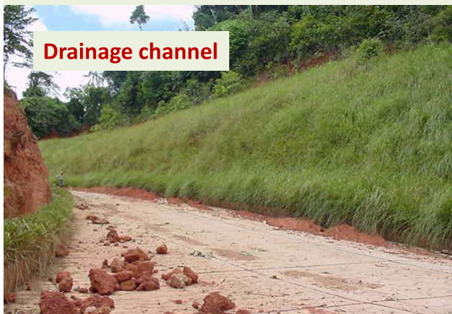
VST for erosion and sedimentation control at Los Pijiguaos Bauxite mine
