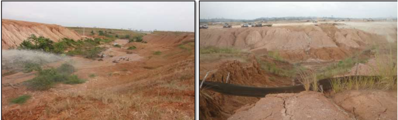
Excessive Erosion Caused by Surface Water Runoff
