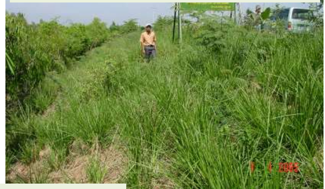
Effectiveness of vetiver planting in protecting dikes from flood erosion
