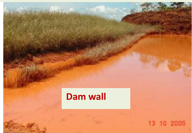
VST for erosion and sedimentation control at Los Pijiguaos Bauxite mine
